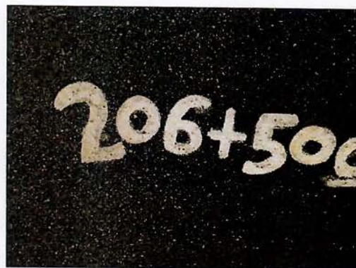
GAC Photos 9: Showing Bleeding along the road corridor from Gharnga to Ganta Guinea Border
