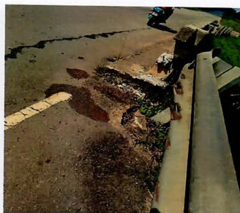
GAC Photo 5c Showing Damage Guardrails and Guardrail with damaged or missing Reflector
