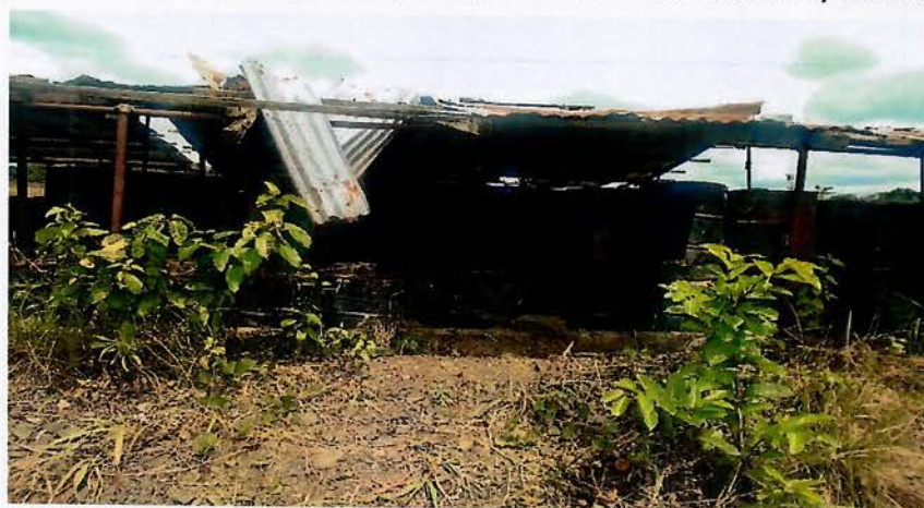
GAC Photo 2c Showing bitumen containers at Weala Quarry Site
