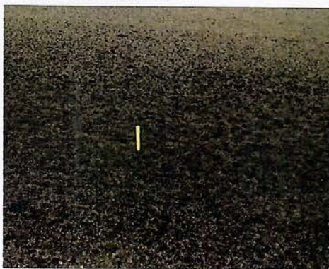
GAC Photos 9: Showing Bleeding along the road corridor from Gharnga to Ganta Guinea Border
