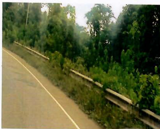
GAC Photo 5c Showing Damage Guardrails and Guardrail with damaged or missing Reflector
