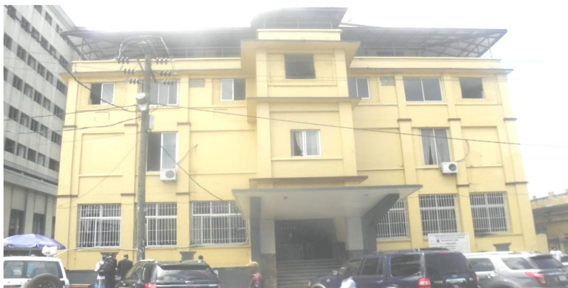
Figure 1: Headquarters of the General Auditing Commission, Ashmun Street, Monrovia, Liberia
