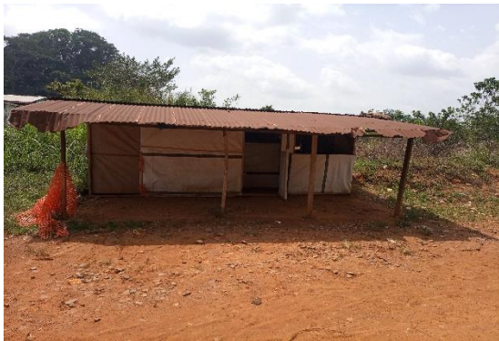
Triage built at yekepa land border Source: GAC Photo 6
