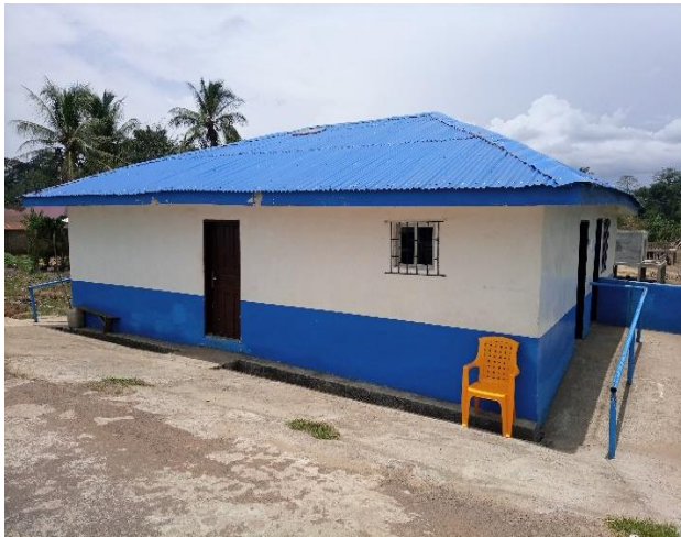
Triage constructed at Bo waterside Source: GAC Photo 4
