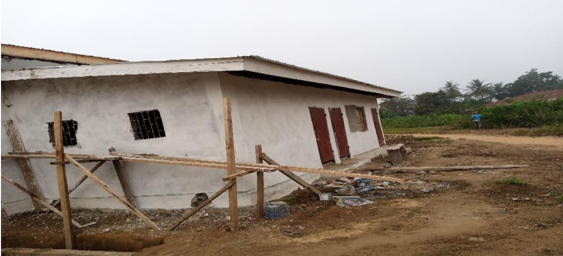
Side View of the Incomplete Warehouse in Karnwee, Saclepea Mah
