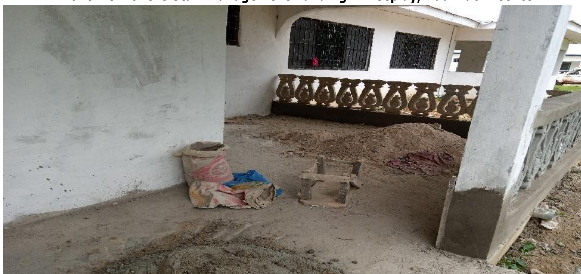
Back View of the Staff Management Building in Beeplay, Buu-Yao District
