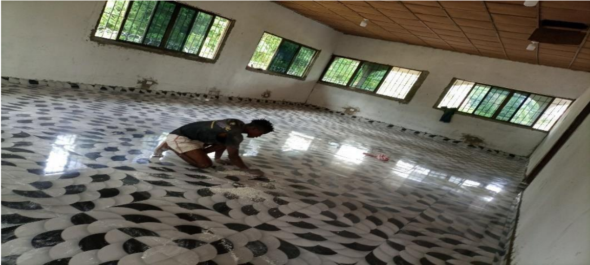
Interior of the Staff Management Building in Beeplay, Buu-Yao District
