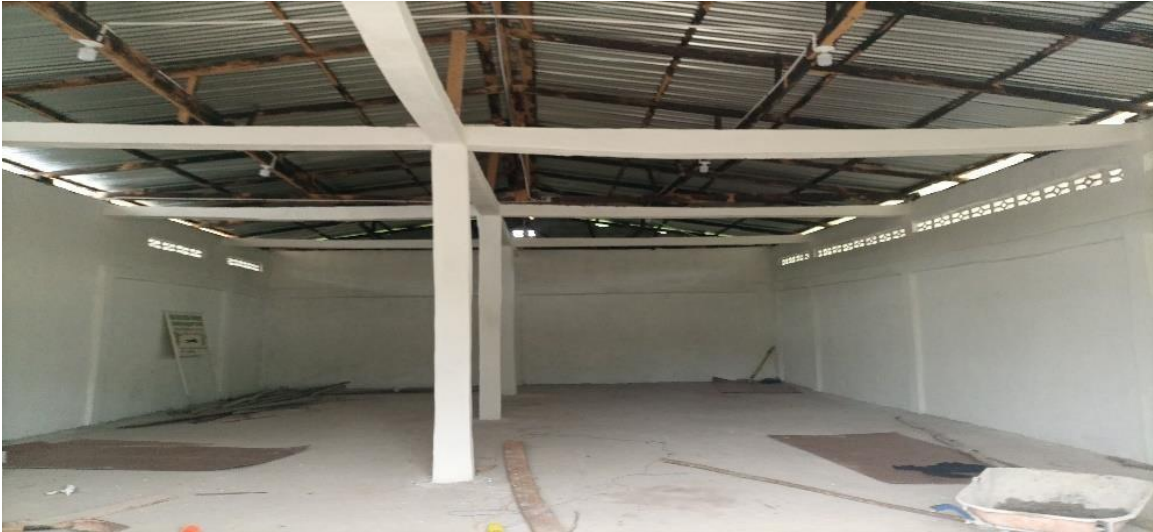
Interior of Incomplete Warehouse in Bloulay, Buu-Yao District
