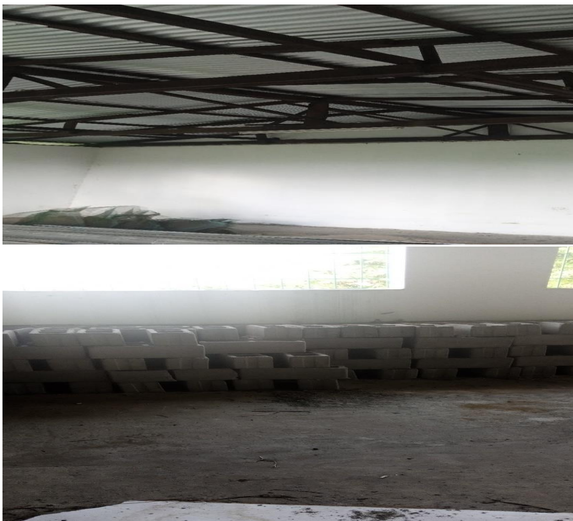
Interior view of MoA warehouse in Buchanan city, Grand Bassa County
