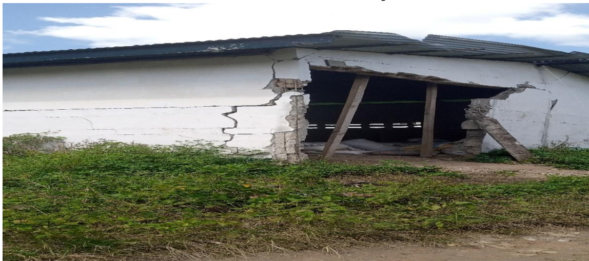
Back view of MoA warehouse in Voinjama city, Lofa County
