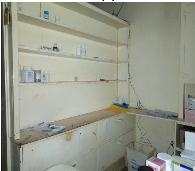
Liberia Government Hospital dispensary
