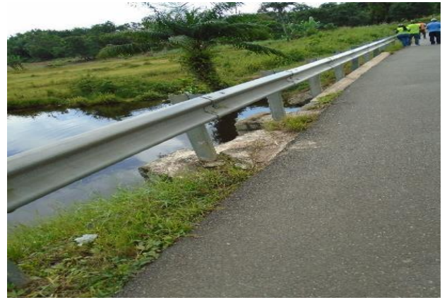
GAC Photos 7: Showing Damaged reflectors and Guardrail with no reflectors on Monrovia to Gbarnga road corridor
