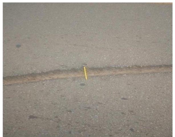
GAC Photo 5: Showing Unrepaired Cuts on Asphalt Pavement, Monrovia to Gbarnga corridor in Lot 1
