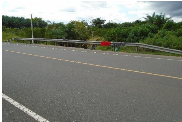
GAC Photos 7: Showing Damaged reflectors and Guardrail with no reflectors on Monrovia to Gbarnga road corridor
