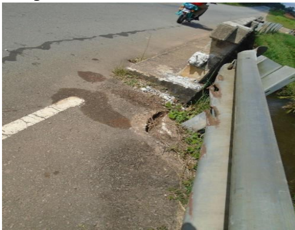
GAC Photos 6: Showing Damage to guardrail along the road corridor from Monrovia to Gbarnga
