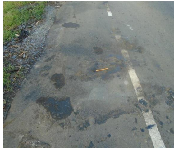
GAC Photo 4: Showing Unrepaired Damaged Access Road and Pavement, Monrovia to Gbarnga corridor in Lot 1
