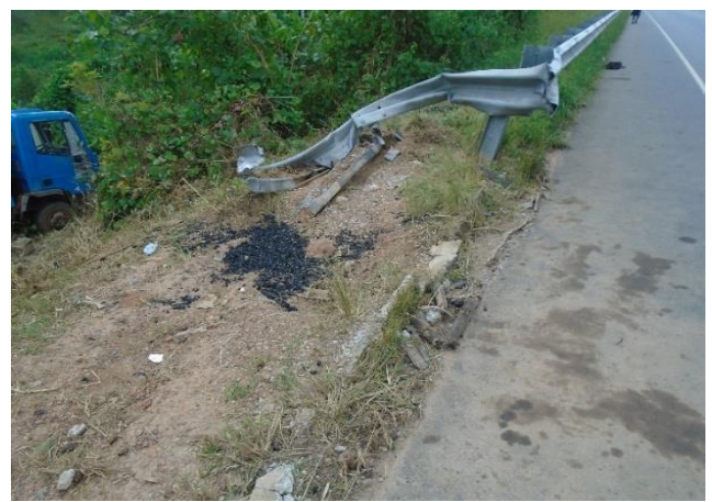
GAC Photos 6: Showing Damage to guardrail along the road corridor from Monrovia to Gbarnga
