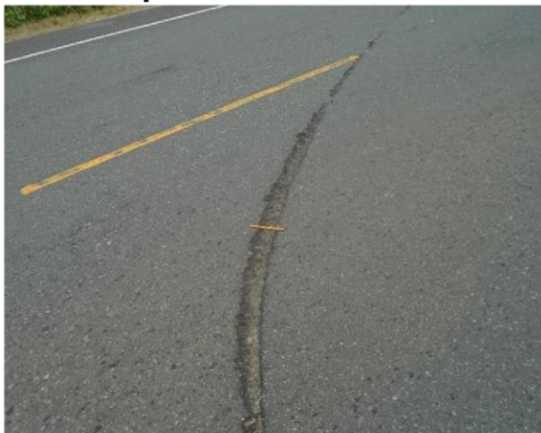
GAC Photo 5: Showing Unrepaired Cuts on Asphalt Pavement, Monrovia to Gbarnga corridor in Lot 1
