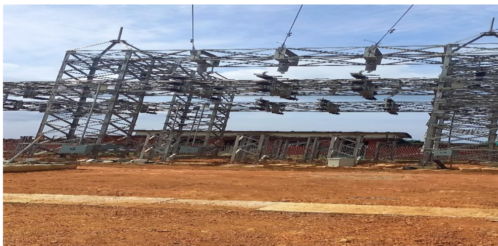
GAC photo: Stockton Creek Substation in the Slaughterhouse Community
