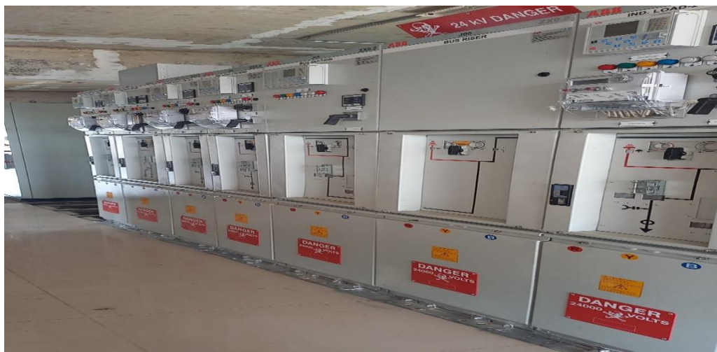
GAC photo: Stockton Creek Substation Control room installation in progress
