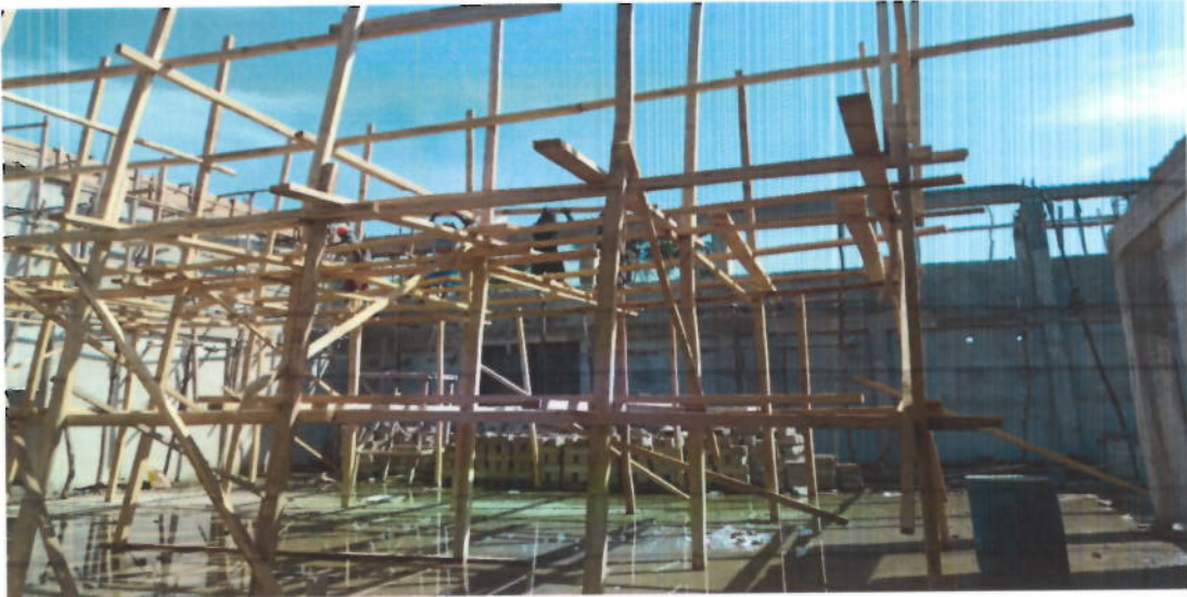
Unfinished Substructure Interior view 3
