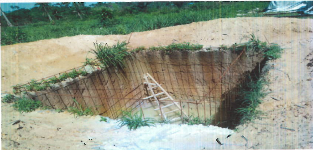
Uncompleted Septic Tank
