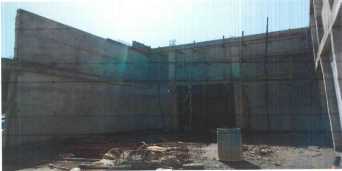
Unfinished Substructure Interior View -1
