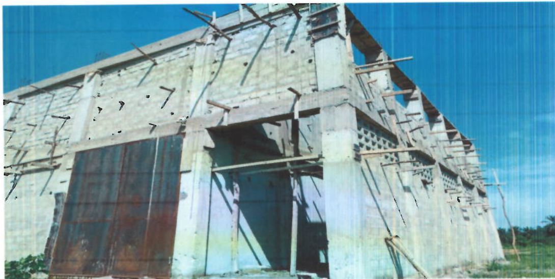
Unfinished Substructure View 1
