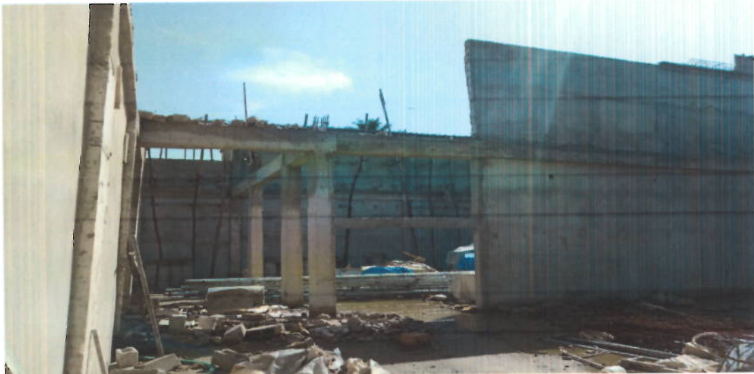
Unfinished Substructure Interior View 2
