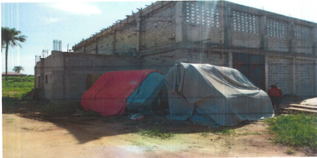
Equipment (Rice Milling) outside Structure
