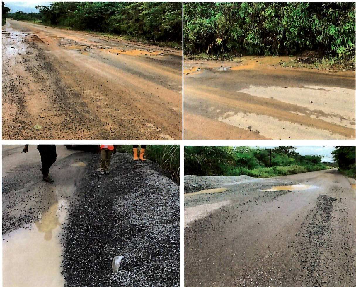
GAC Picture 3 showing potholes and damaged asphalt on the carriageway from St. Paul to Bo-Waterside Road Corridor
