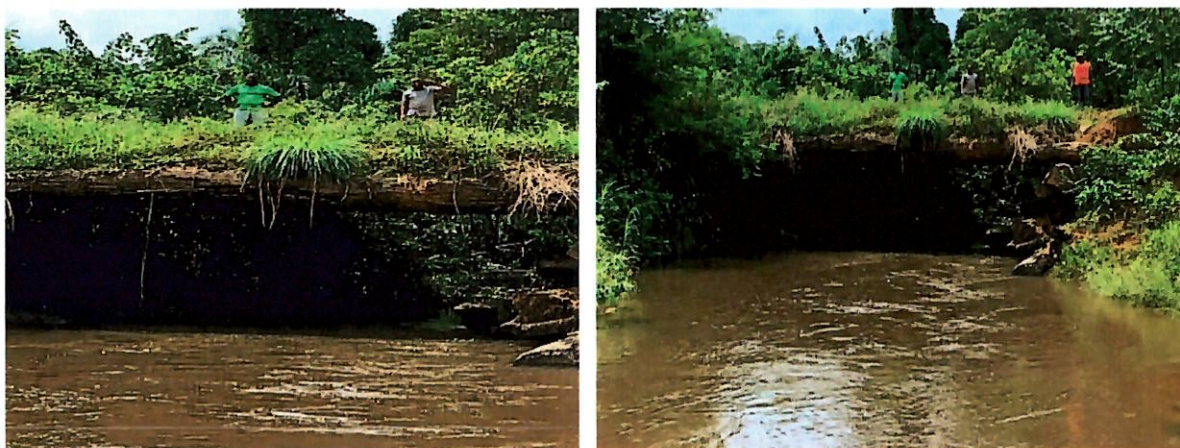
GAC Picture 2 showing a log/timber bridge over the Weagbeh River to Jennemaneh Township
