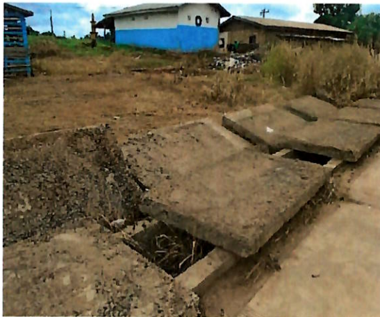
GAC Picture 11 showing incomplete concrete side drains that are yet to receive concrete slabs/covers on the Gbarnga Broad Street.
