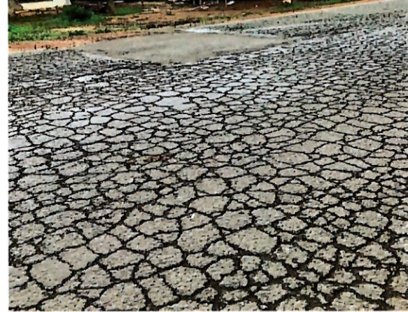
GAC Picture 4 showing alligator cracking and potholes along the Klay to Tubmanburg Road corridor in Bomi County
