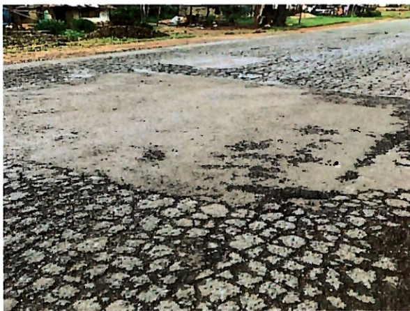
GAC Picture 4 showing alligator cracking and potholes along the Klay to Tubmanburg Road corridor in Bomi County
