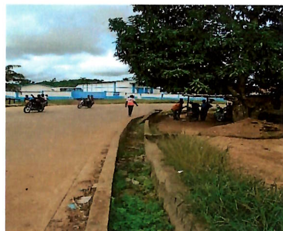
GAC Picture 11 showing incomplete concrete side drains that are yet to receive concrete slabs/covers on the Gbarnga Broad Street.
