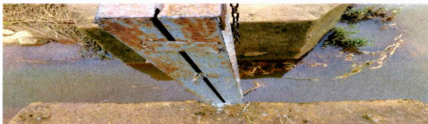
Damage gate of the peripheral canal
