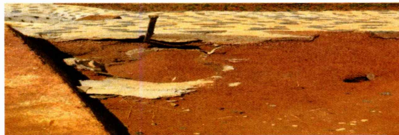
The Embankment of the Reservoir is not stone Pitch and the Embankment is sinking
