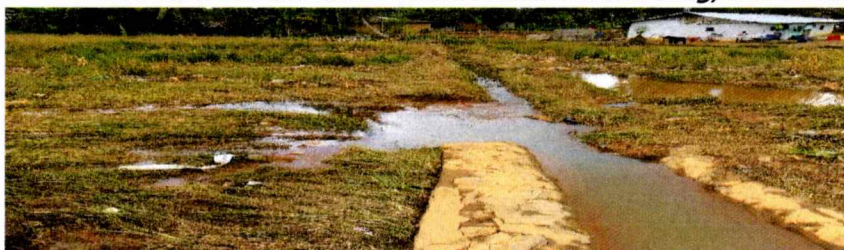
Flooding from the community into the peripheral canal destroying the Layout
