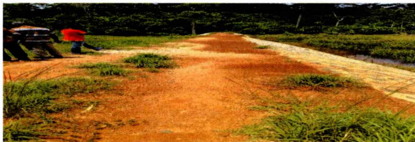
The Embankment of the Reservoir is not stone Pitch and the Embankment is sinking
