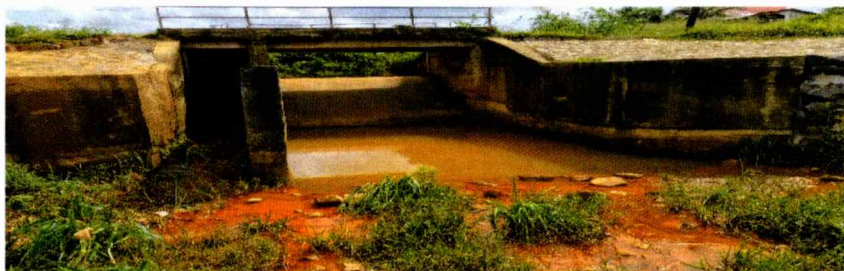
The reservoir for both Pleebo A and B is not drag, and there is no water
