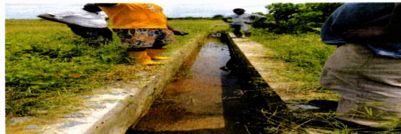
The Central Canal is Cast (cement without stone), and the abandonment of farmland by farmers
