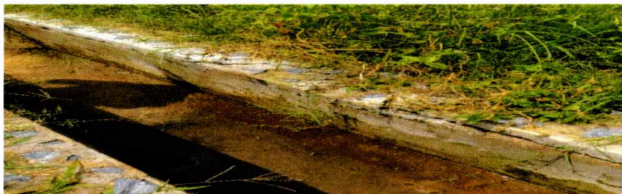
The Peripheral Canal is built with cement blocks, and a portion of it is destroyed by erosion
