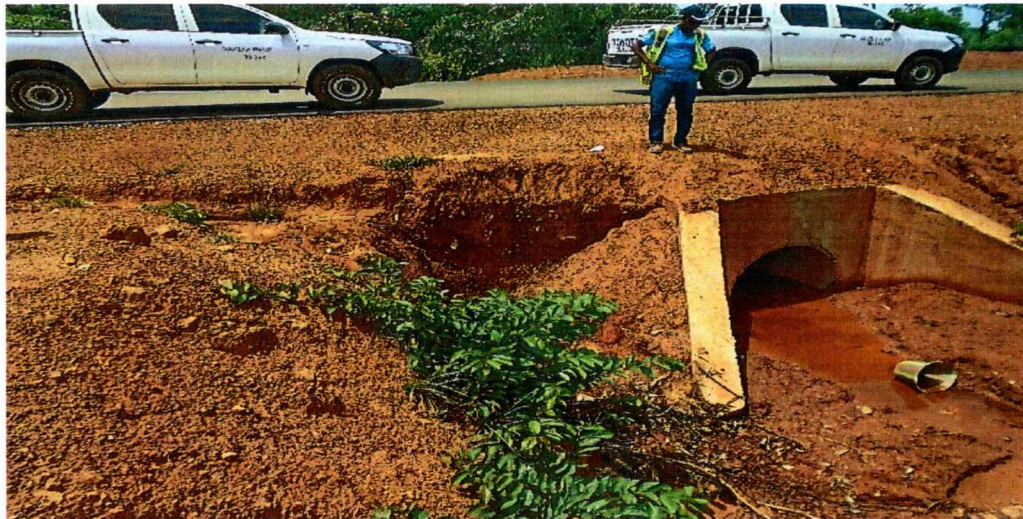
GAC photo 3: Showing sections that needed grass planting to protect a streambank from erosion
