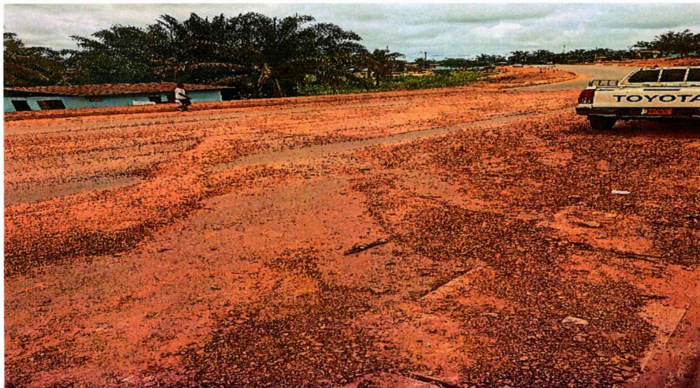
Photo 6: Showing Erosion, sand/debris
