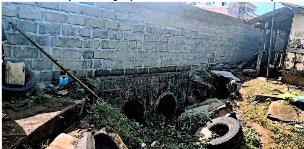
EXHIBIT 8: GSA Road Drainage System
