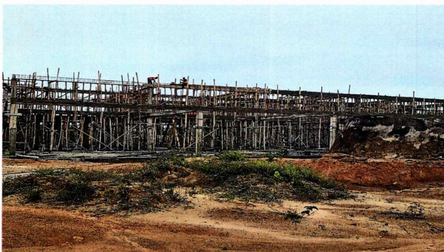
GAC: A partial view of the uncompleted Karnplay Market in May 2025
