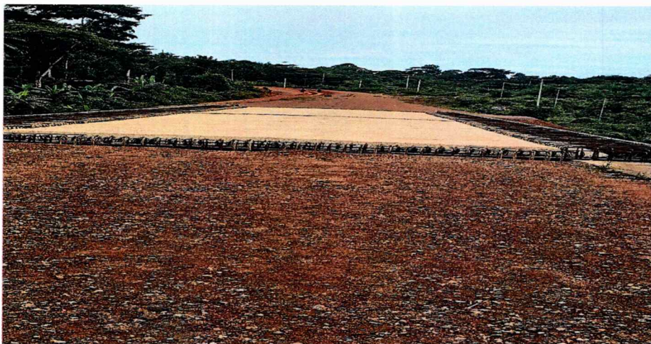
GAC Photo: A partial view of the suspended road construction project (Sanniquelle to Loguatu road 47.1km)
