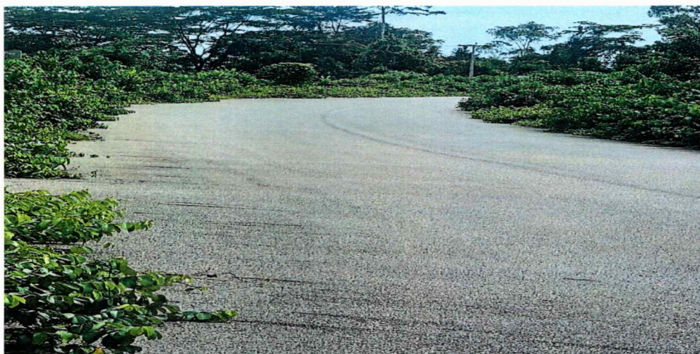
GAC: Partial view of the abandoned Karloken to Fishtown road (80km)
