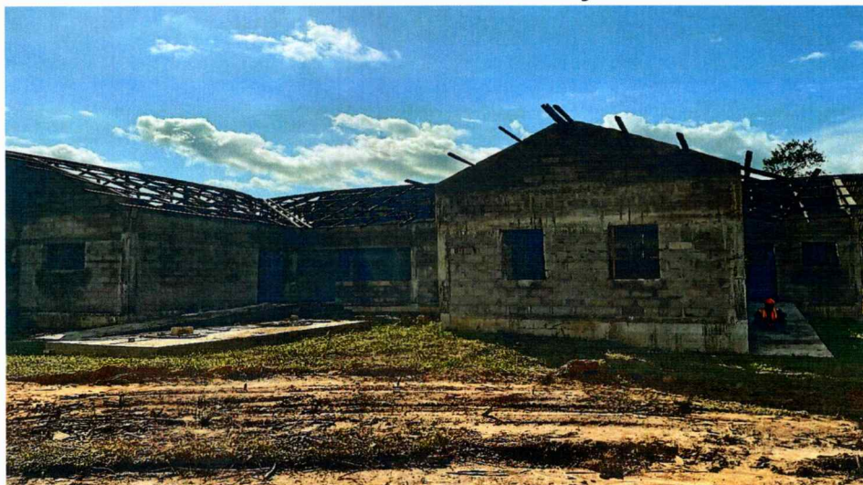
GAC Photo 12: Exterior View of Bambuta Construction Project in Gbarpolu
