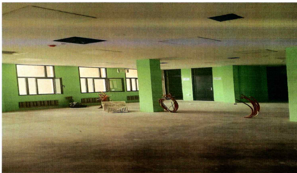
GAC Photo 3: Uninstalled Medical Equipment at the NRH
