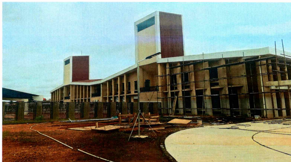
GAC Photo 6: Exterior View of the New Redemption Hospital
