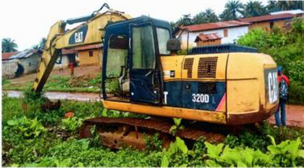
Crawler Track Excavator (320DL - KGL-061338), Location - LPMC Compound
