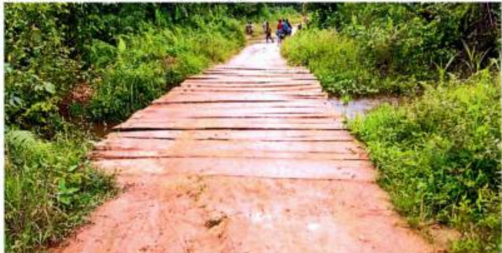
Construction of Bridges, Cost US$ 20,000.00, in District No. 8; Kpein, Zekepa Town, Zehnlá; Contractor: Focus Construction and Architectural Company
