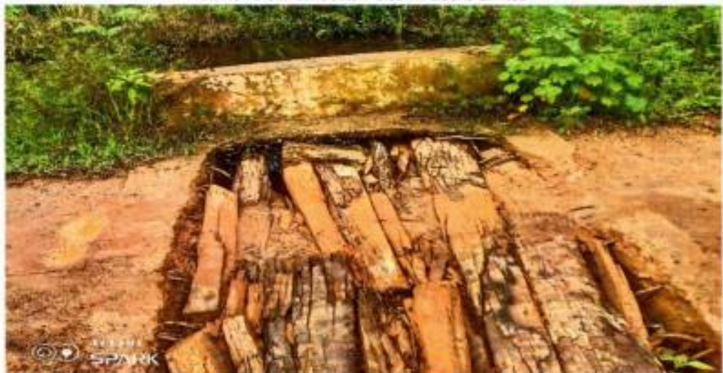
Construction of Bridges, Cost US$20,000.00 in District No. 7; Zoe Clans, Gbao, Wee Gbehyi (Fleedin to Forkoleh River). Contractor: Atlantic Engineering and Construction Company Limited
