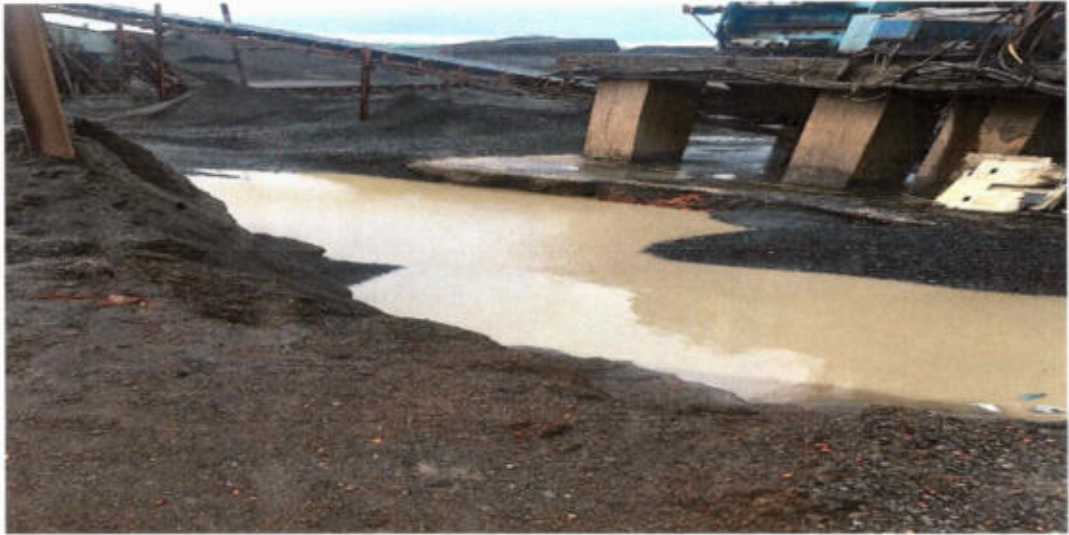
GAC Photo 3a: Showing a direct discharge of sanitary or wash water from the quarry, batching, and asphalt plants to surface water
