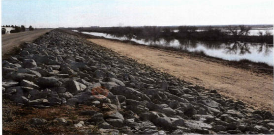
GAC photo 1a: Showing examples of Riprap protection and Riprap used to protect a streambank from erosion
