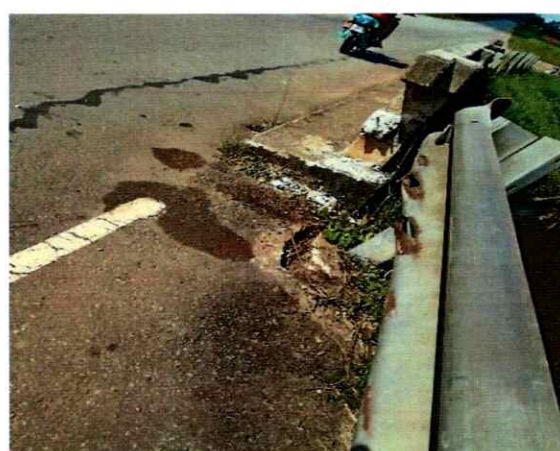
GAC Photo 7c Showing Damage Guardrails and Guardrail with missing Reflector
