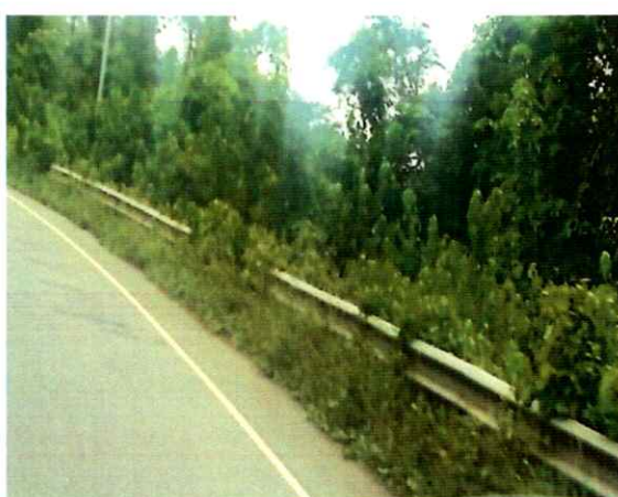
GAC Photo 7c Showing Damage Guardrails and Guardrail with missing Reflector
