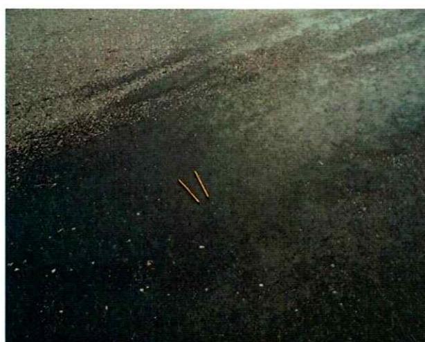
GAC Photos 4 Showing Bleeding Asphalt on Pavement Surface, Monrovia to Gbarnga corridor in Lot 1
