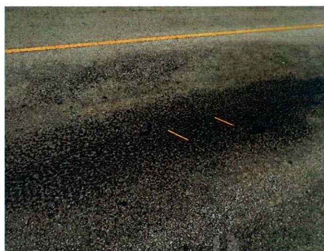
GAC Photos 4 Showing Bleeding Asphalt on Pavement Surface, Monrovia to Gbarnga corridor in Lot 1
