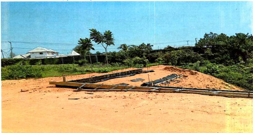
GAC Photo 3: Foundation for medical waste under construction at the NRH
