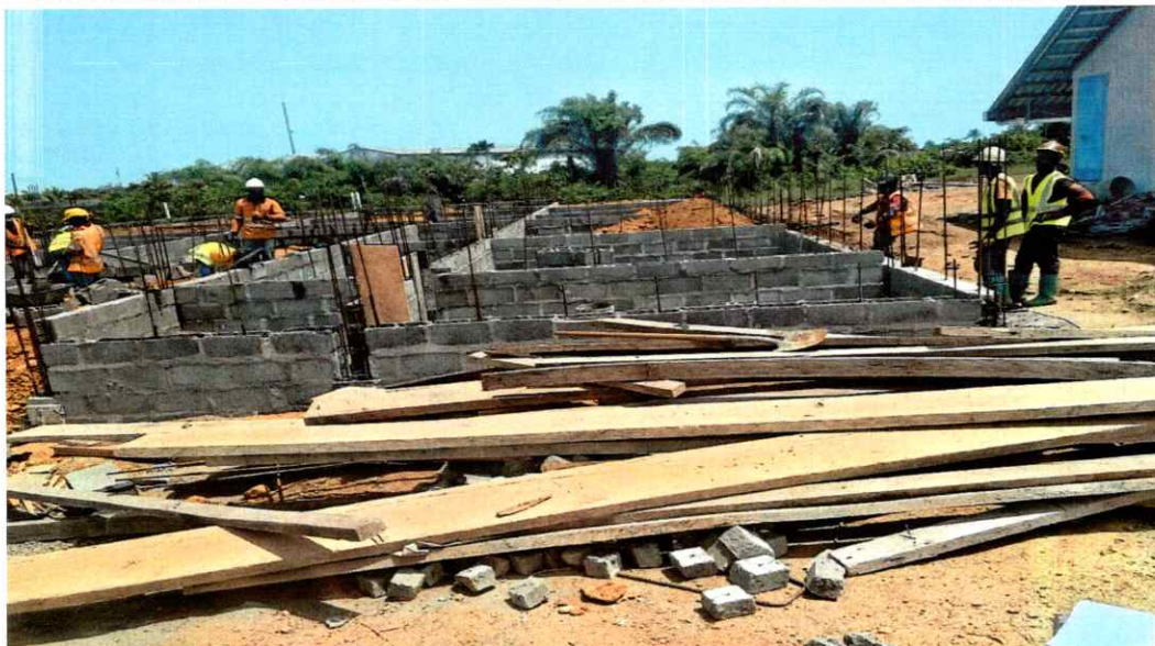
GAC Photo 3: Foundation for medical waste under construction at the NRH
