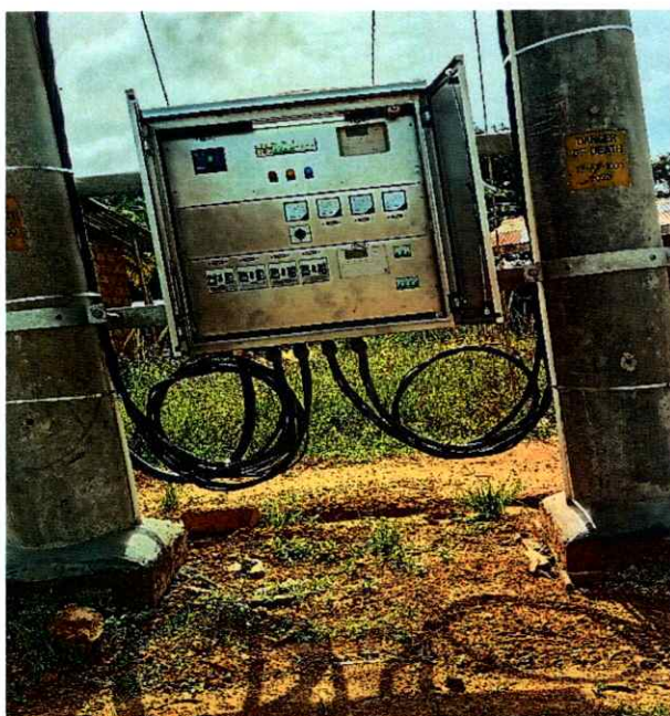
Transformer Meter Board - Rivercess at the Yarpah Town 1 General Hospital, River Cess County
