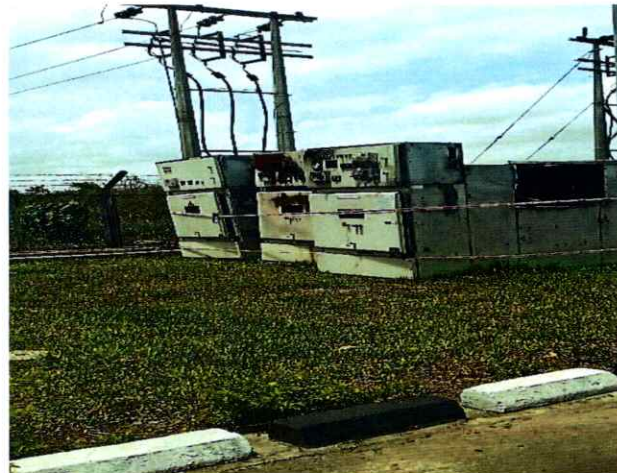
The feeder boxes that destroyed by fire in the control room at the RIA substation
