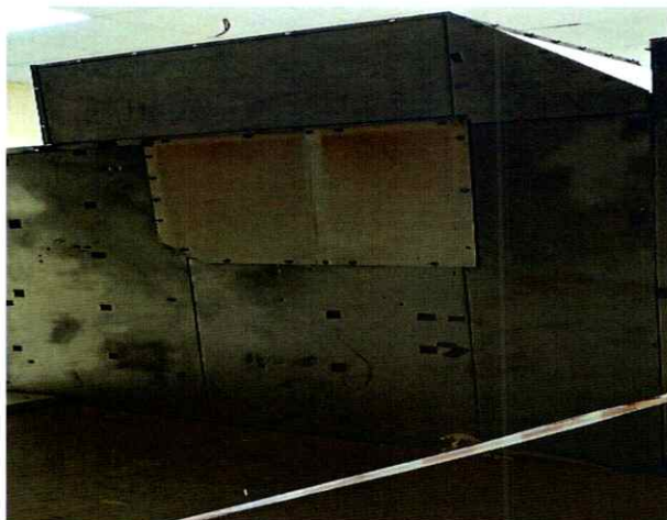
The feeder boxes that destroyed by fire in the control room at the RIA substation
