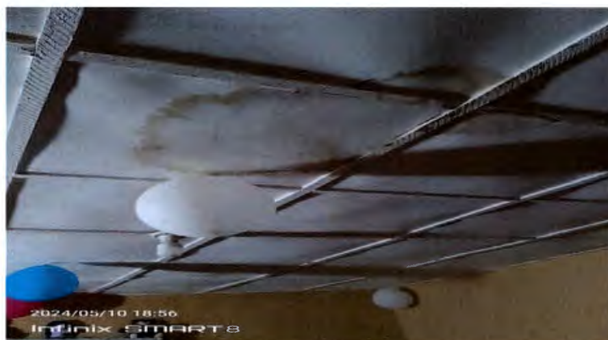
Bopolu City, Gbapolu County Staff Housing Unit leakage problem
