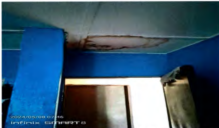
Partial view of Rivercess Staff Housing Units leakage problem
