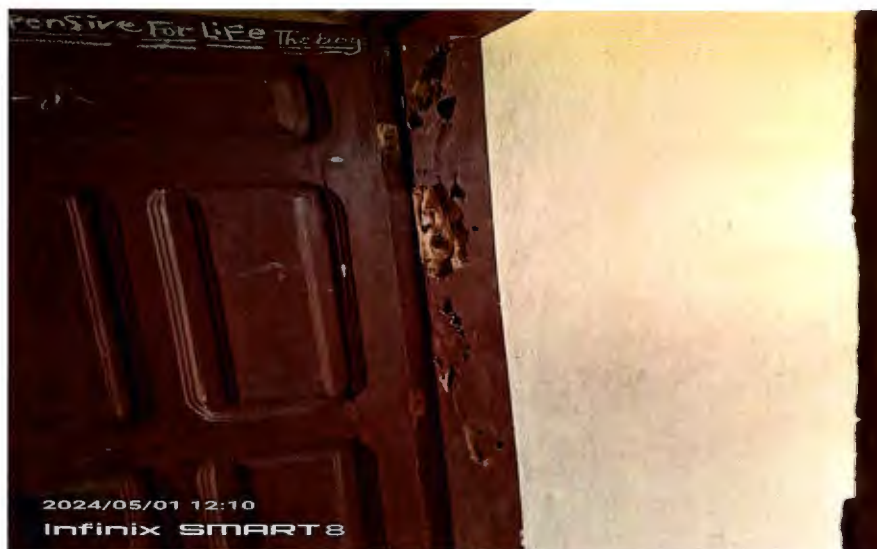
Rivergee County Staff Housing Units Door Frame eating by termites
