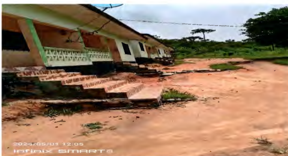
Partial front View of Rivergee County Staff Housing Units steps undermine by erosion
