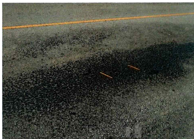
GAC Photos 3 Showing Bleeding Asphalt on Pavement Surface, Monrovia to Gbarnga corridor in Lot 1
