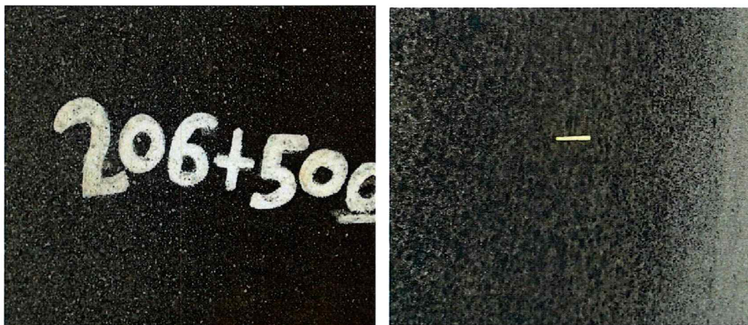
GAC Photos 9: Showing Bleeding along the road corridor from Gharnga to Ganta Guinea Border
