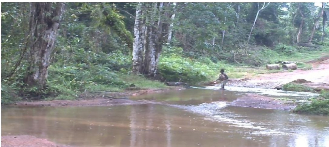
Figure 2 A view of a segment of the Nyonbeh Town-Wheasaye (Grand Kola) road awaiting the installation of culverts.
