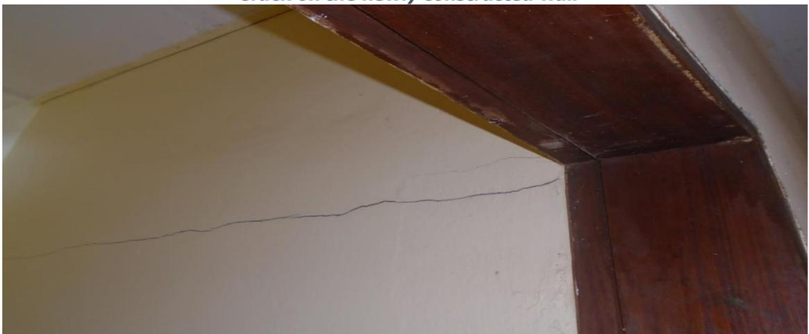
***Crack over the door frame***
