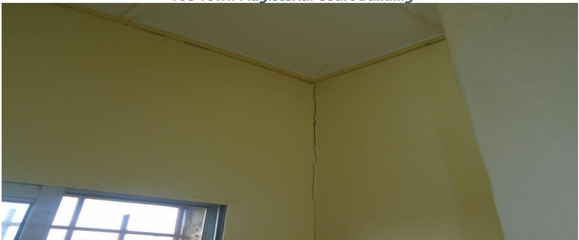
***Crack on the newly constructed wall***
