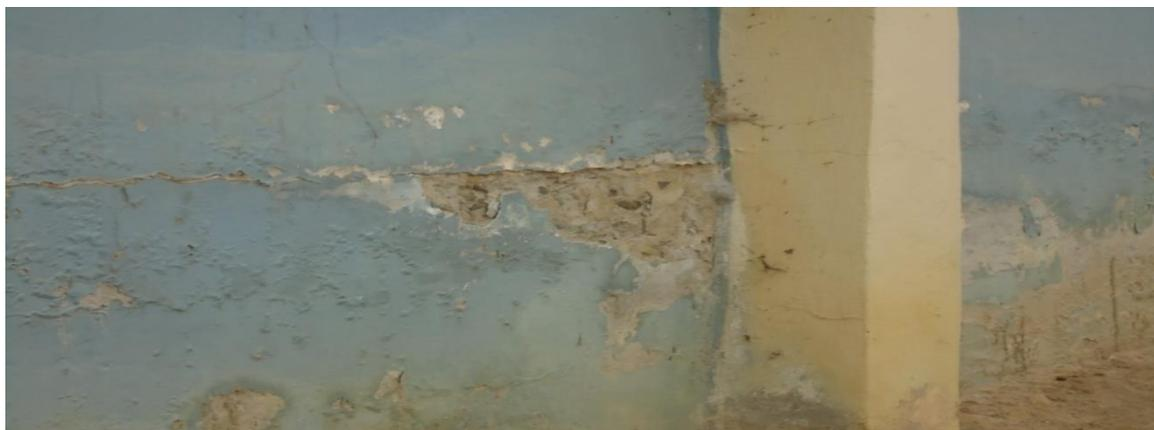
**GAC Photo 1: Crack on the newly constructed Foundation**
