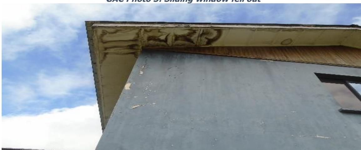
**GAC Photo 4: Leaking Roof**
